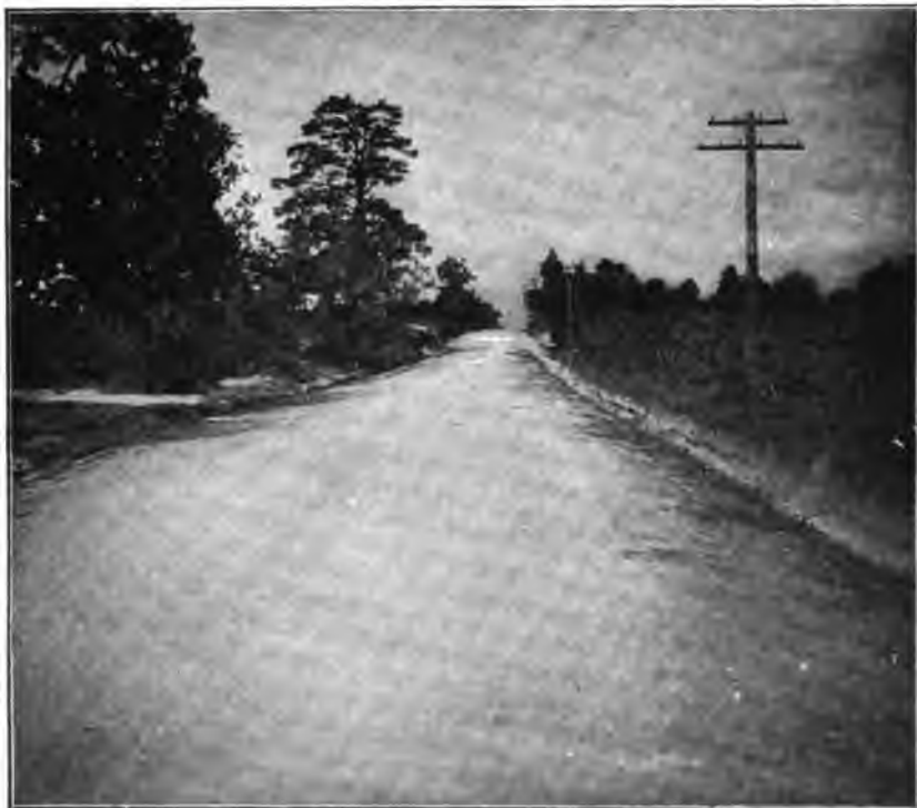
A COMPLETED SAND-CLAY ROAD.
